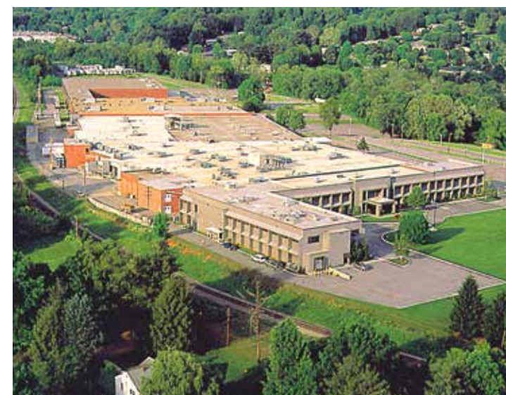
AERUS MANUFACTURING PLANT | BRISTOL, VA
